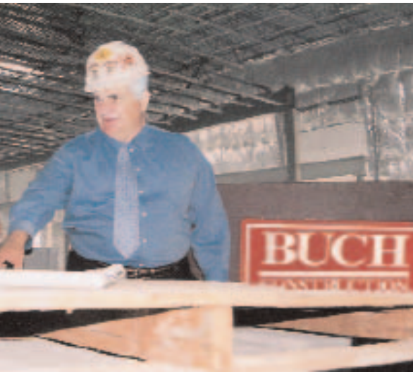
MARCC CEO/EST Bill Halbert (right) discusses building plans with Seldon Taylor, Buch Construction company site superintendent.
